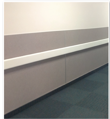
After: Allure panels installed directly over rigid plastic panels.
