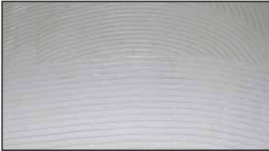
Example of properly troweled adhesive application
